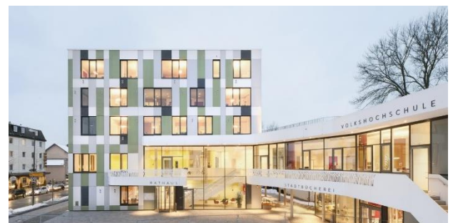
Figure 3 Townhall of Kolbermoor
